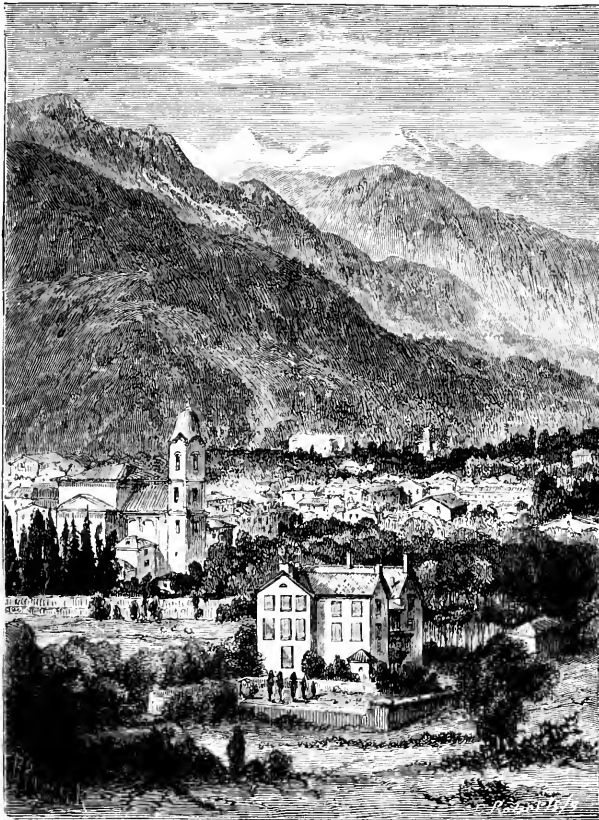
GENERAL VIEW OF LA TORRE.
