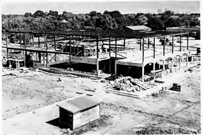
131. Construction of Hamman Hall, 1957.
