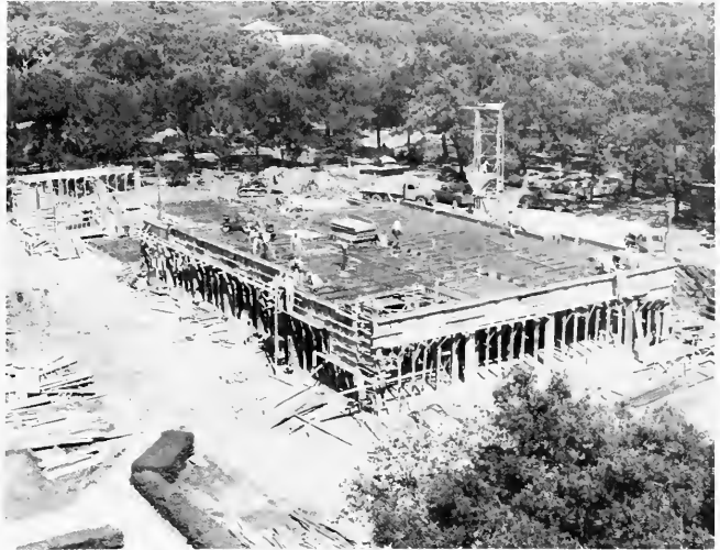
145. Rayzor Hall during construction, May 10, 1961.
