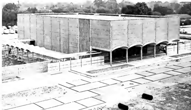
132. Hamman Hall, a view of the nearly completed building, April 14, 1958.
