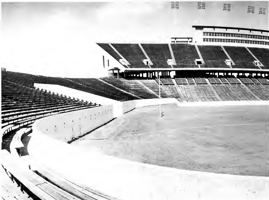
122. Construction of the new Rice Stadium, May 23, 1950.
