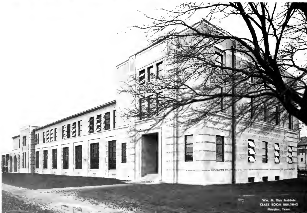
114-116. Construction of Anderson Hall. 114. November 6, 1946. 115. July 1, 1947. 116. December 8, 1947.
