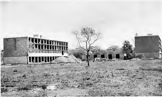
137. Construction of Mary Gibbs Jones College, March 5, 1957.
