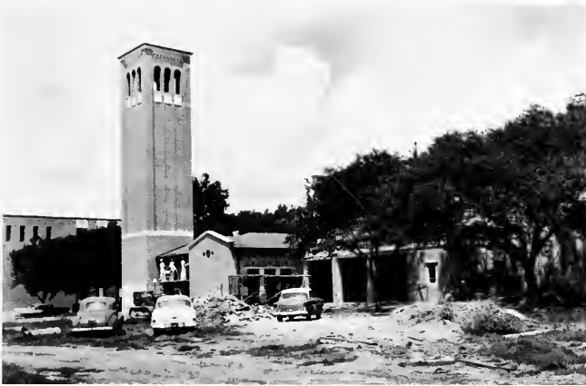
134. Construction of the Rice Memorial Student Center.
