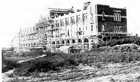
16. Construction of the Administration Building, May 1912.
