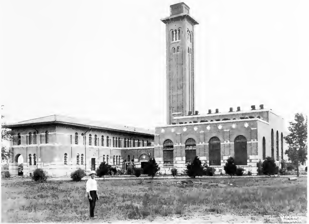
25. The completed Mechanical Engineering Laboratory with landscaping. "Mr. Dennis" is in the foreground.
