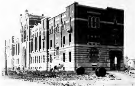
17. The nearly completed Administration Building.
