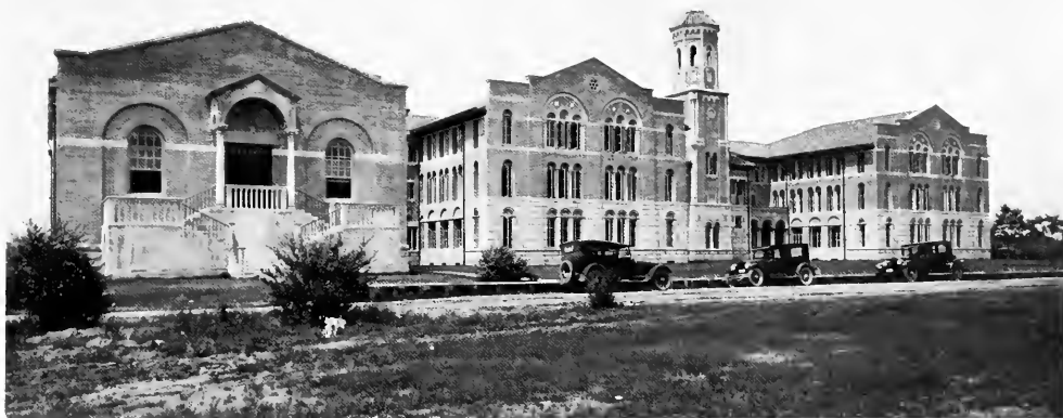
72. Exterior view of the new Chemistry Building, April 28, 1926.
