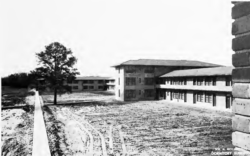
139. Wiess College, construction substantially completed, January 3, 1950.
