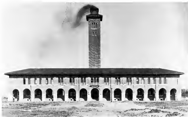
24. Construction photograph of the Mechanical Engineering Laboratory and powerhouse, probably 1912.
