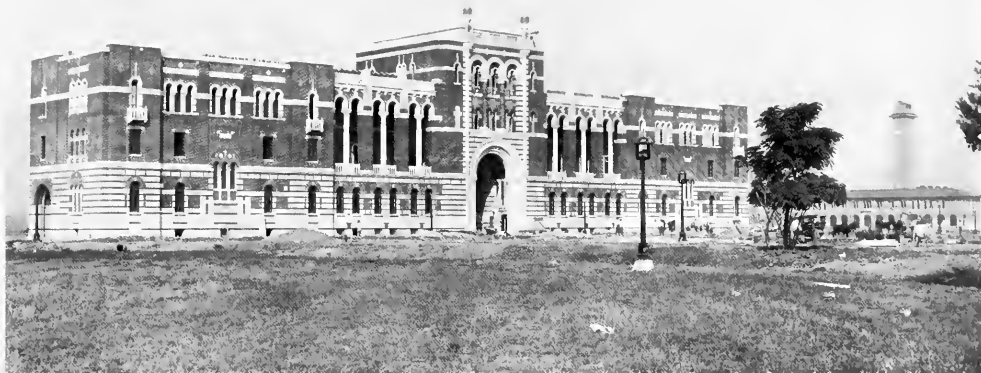
18. The finished building, showing the Mechanical Laboratory to the right.
