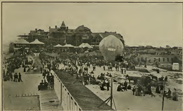
HOTEL DEL CORONADO DURING CONSTRUCTION
