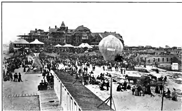
HOTEL DEL CORONADO DURING CONSTRUCTION
