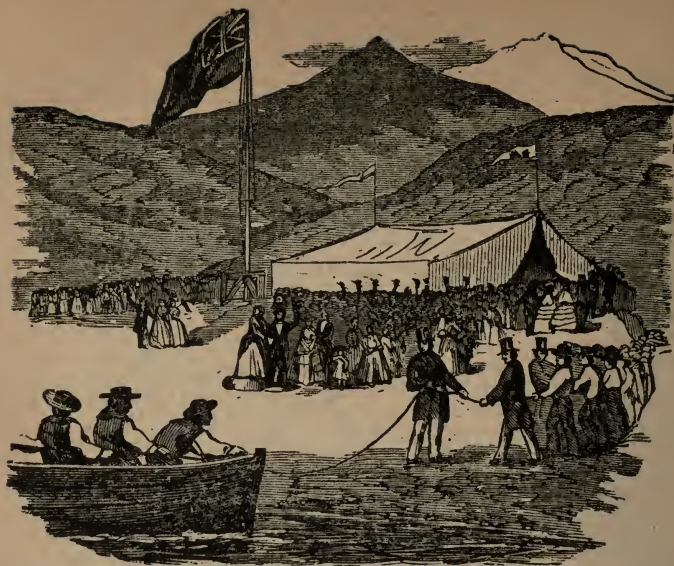
LANDING THE CABLE.
