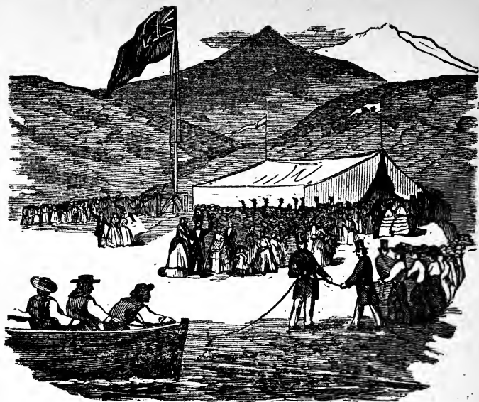
LANDING THE CABLE.
