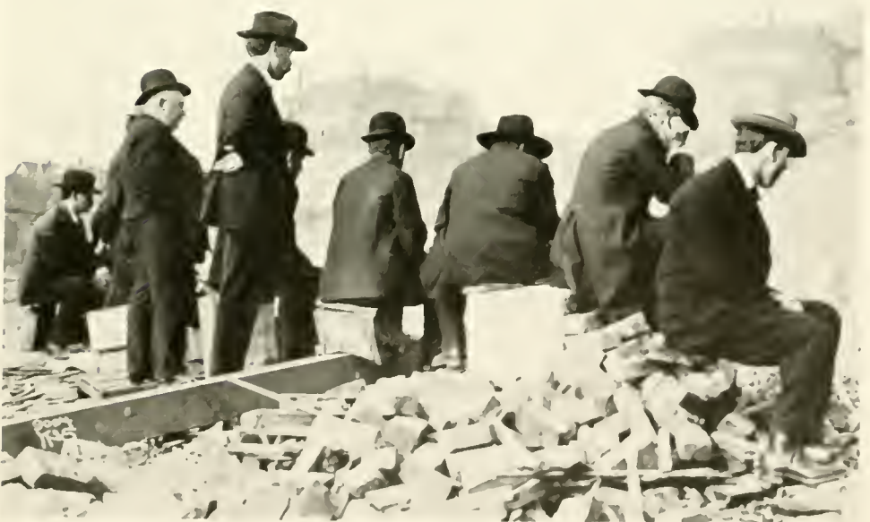
INTEREST IN THE SLICING WORK WAS UNCEASING
