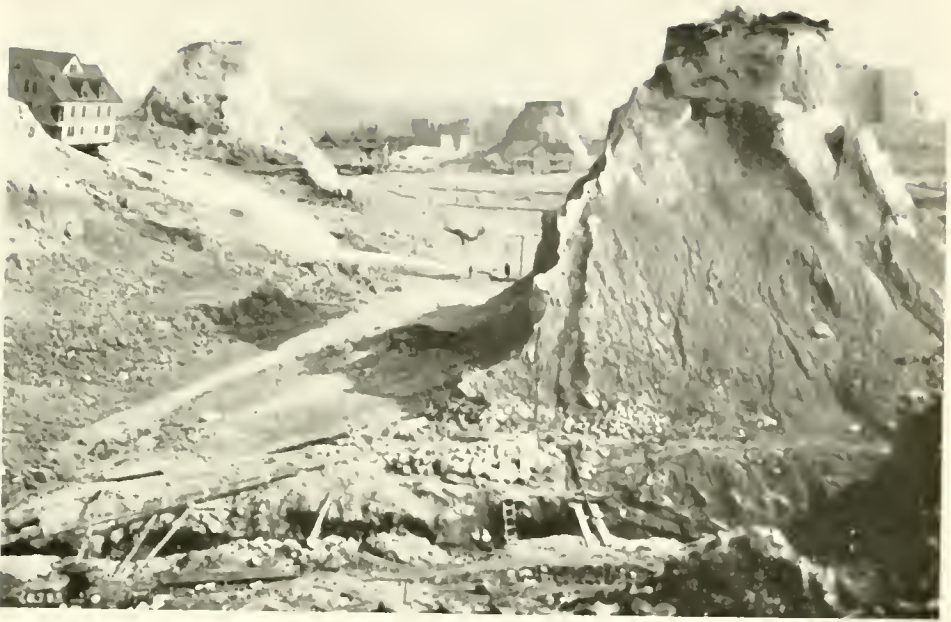
THE DENNY HILL REGRADE NEARING COMPLETION
