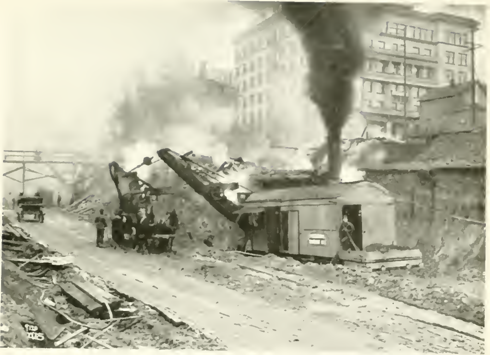
THIRD AVENUE REGRADE AT MARION STREET
