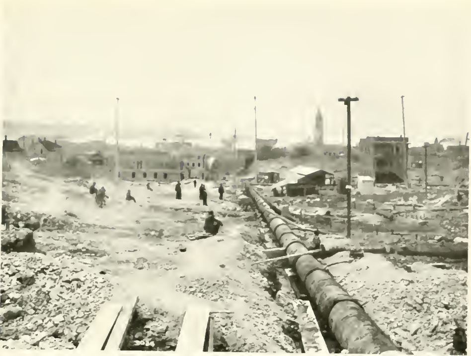
JACKSON STREET REGRADE LOOKING WEST
