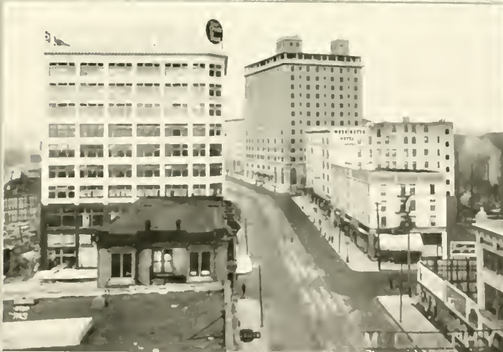
REGRADED AND REBUILT IN THREE YEARS
