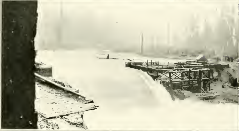
CEDAR LAKE DAM, WITH 5 FEET OF WATER OVER CRACK
