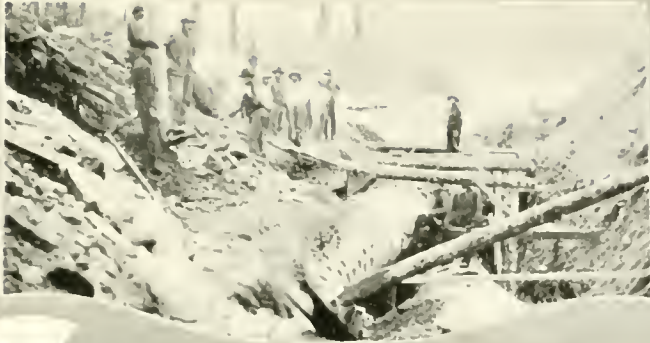
WORKING ON THE DAM
