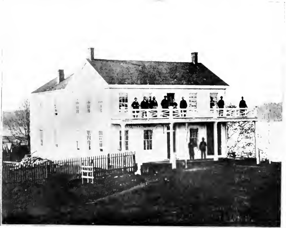
THE FELKER HOUSE, JACKSON STREET AND WESTERN AVENUE
