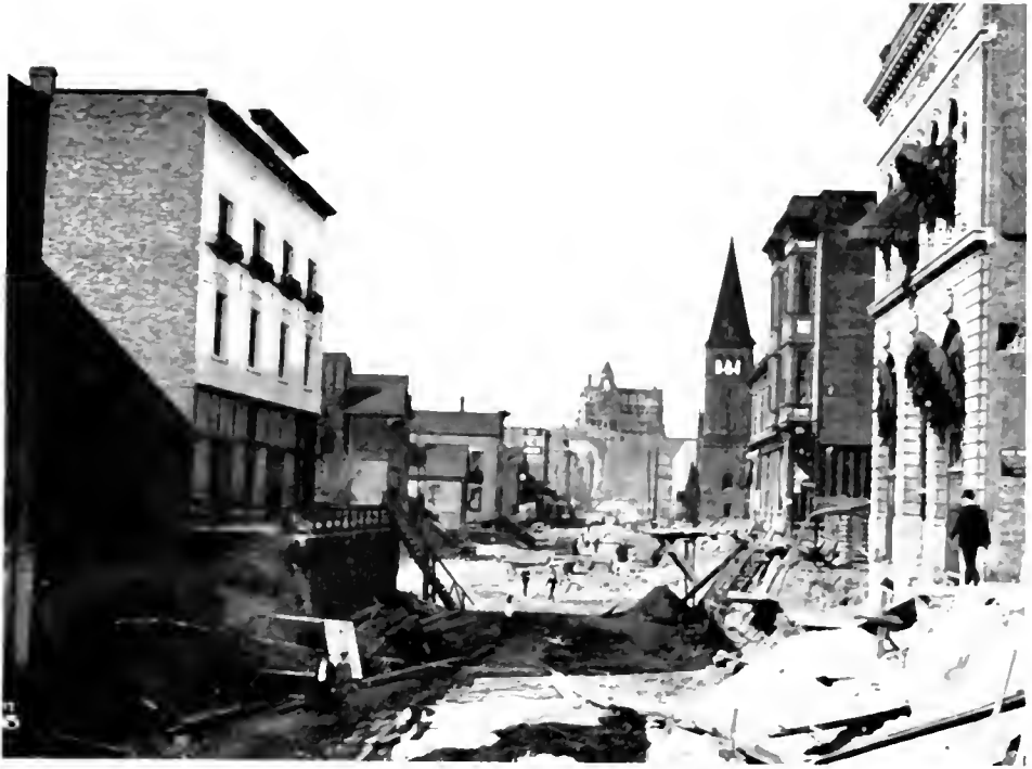
THIRD AVENUE REGRADE NORTH OF SENECA STREET
