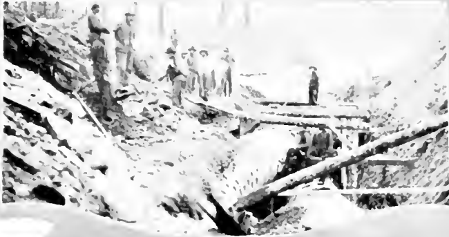
WORKERS ON DAM
