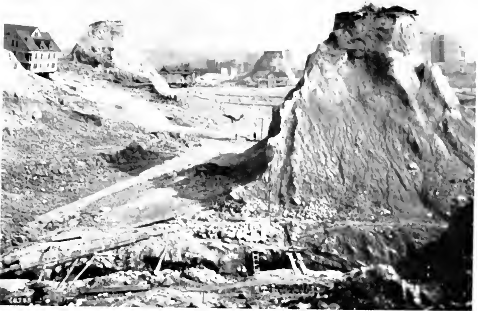
THE DENNY HILL REGRADE NEARING COMPLETION
