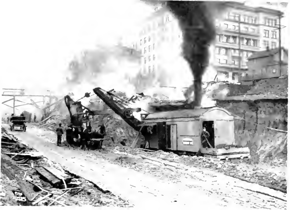
THIRD AVENUE REGRADE AT MARION STREET
