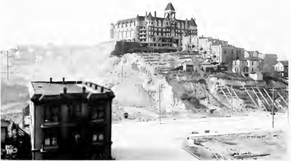
THE SAME BUILDING AFTER SECOND AVENUE WAS CUT DOWN
