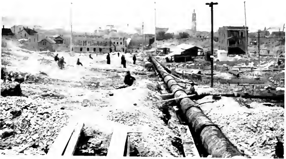
JACKSON STREET REGRADE LOOKING WEST
