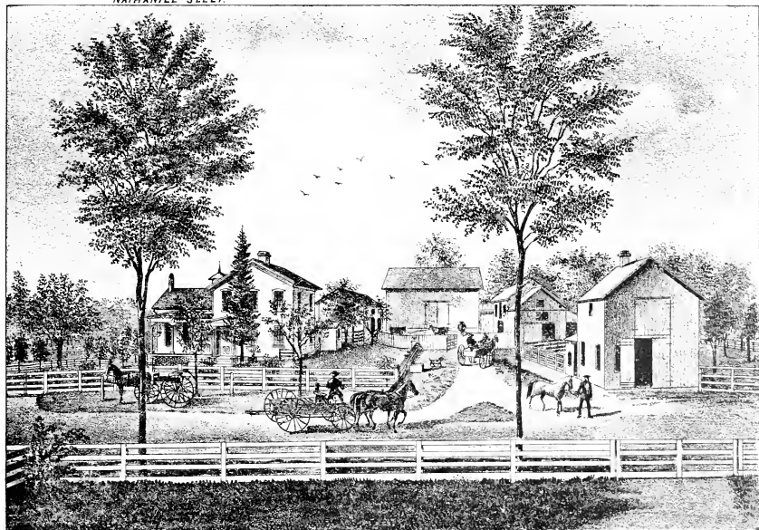
RES. OF NATHANIEL SEELY, BUILDING MOVER. WATERLOO, N.Y.
