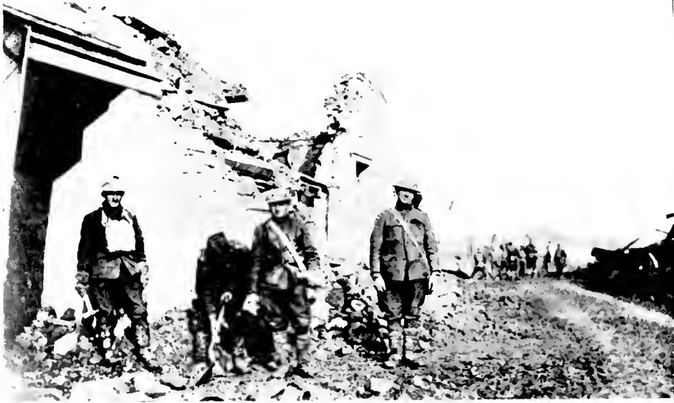
MEN OF THE 304TH ENGINEERS REPAIRING ROAD IN DAMVILLIERS. MACHINE GUN BULLETS WERE CRACKING OVER THEM WHEN THIS VIEW WAS SNAPPED
