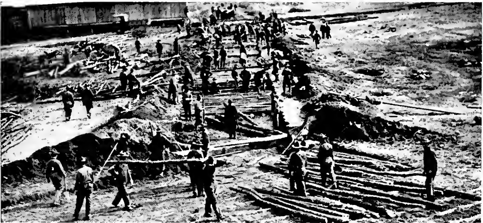
EMERGENCY ROAD CONSTRUCTION BY THE 304TH ENGINEERS AT CAMP MEADE
