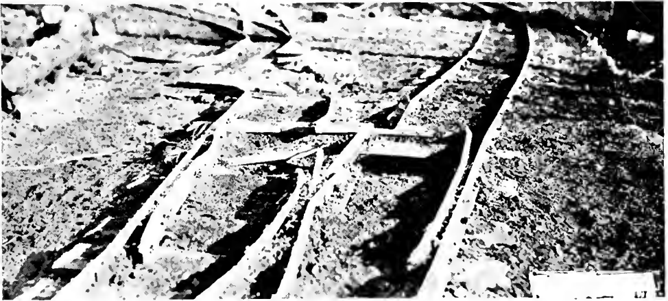
BROKEN RAILROAD TRACKS NEAR MOLLEVILLE FARM.
