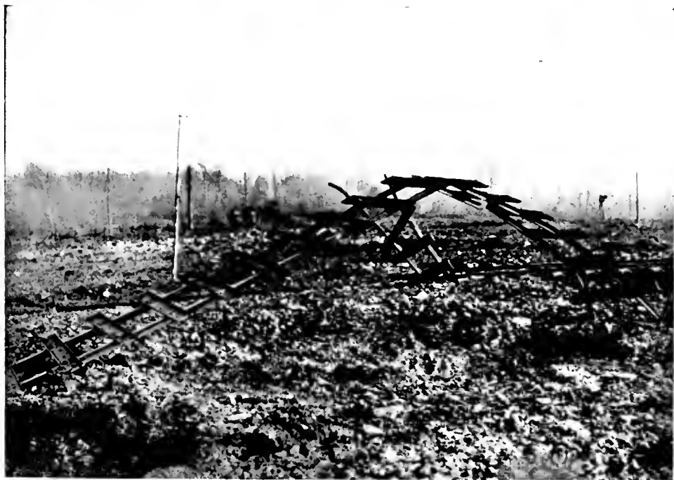
BOCHE NARROW GAUGE RAILROAD AT MOLLEVILLE FARM BLOWN INTO ARCH BY FORCE OF SHELL EXPLOSION.
