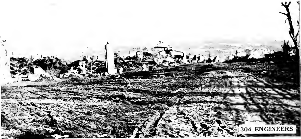
CHARNY, A RUINED TOWN, 7 KILOMETERS NORTH OF VERDUN, USED AS A REGULATING STATION.
