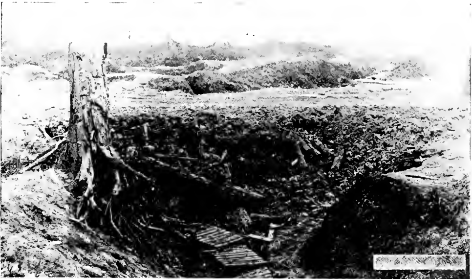
AXIAL ROAD, AVOCOURT—MALANCOURT, SHOWING FILL AT POINT WHERE GERMAN TRENCH CROSSED ROAD.
