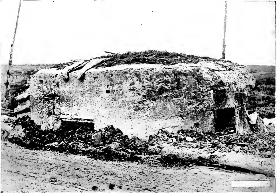
GERMAN PILL BOX ON SLOPE OF MONTFAUCON.
