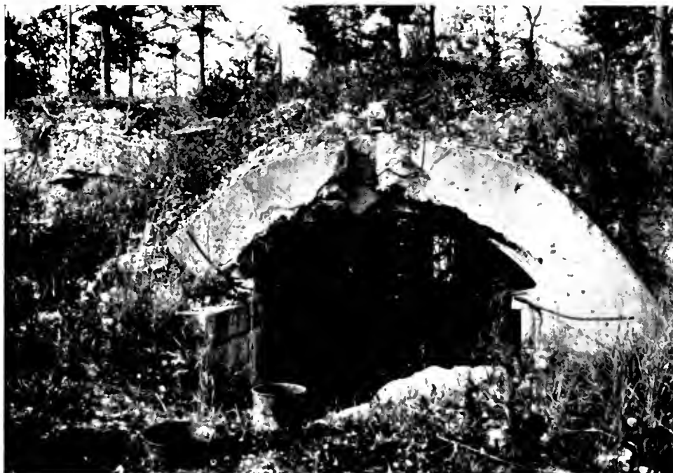
BOCHE CONCRETE SHELTER ALONG ROAD THROUGH BOIS DE CONSENVOYE, NEAR UPPER END OF DEATH VALLEY AND MOLLEVILLE FME.
