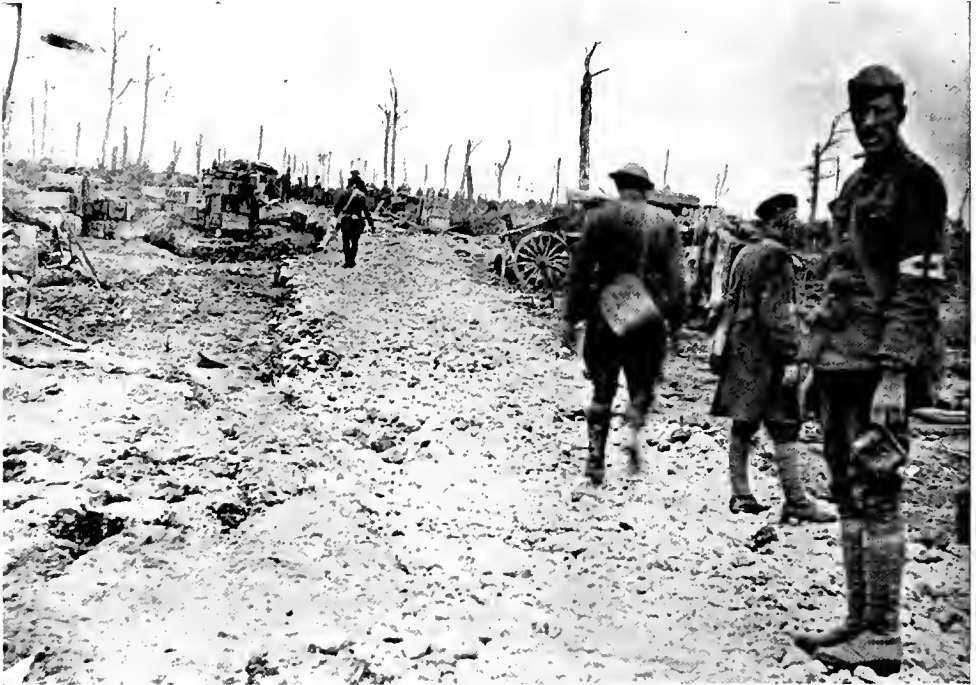
DUMP ON ROAD LEADING FROM AVOCOURT-MALANCOURT ROAD.
