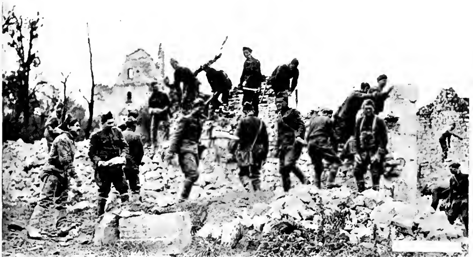
DEMOLISHING WALLS FOR ROAD-BUILDING STONE—ST. REMY-TROYON SECTOR.
