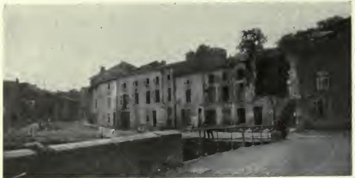
Traffic bridge in the center of the town which was a special artillery target.
