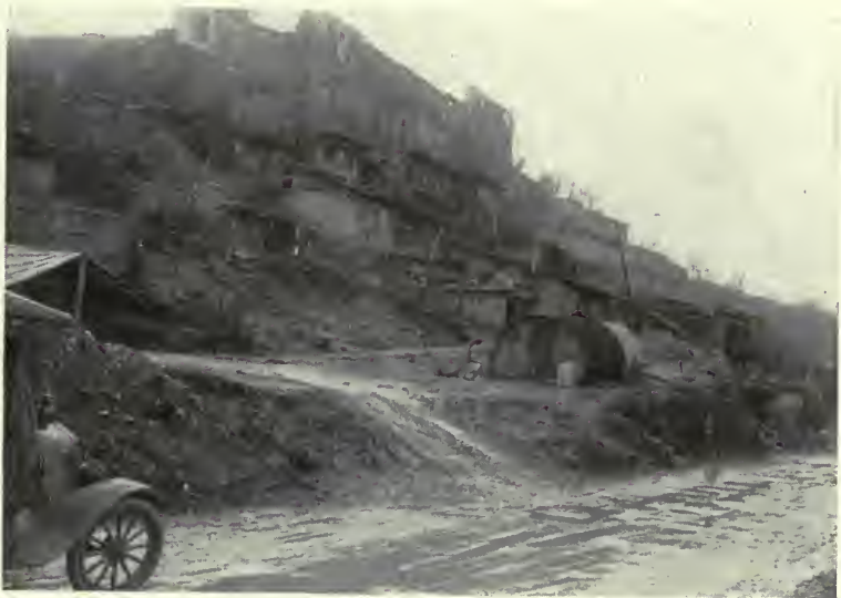
Road leading out of YARBNNES with notable group of German war huts on the hillside.
