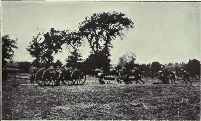
Machine Gun Company training at BOURSIN
