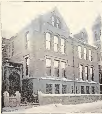
SAMUEL G. HOWE PRIMARY SCHOOL. West Fifth Street.
