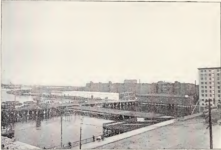
CONGRESS STREET BRIDGE. (From roof of South Union Station.)
