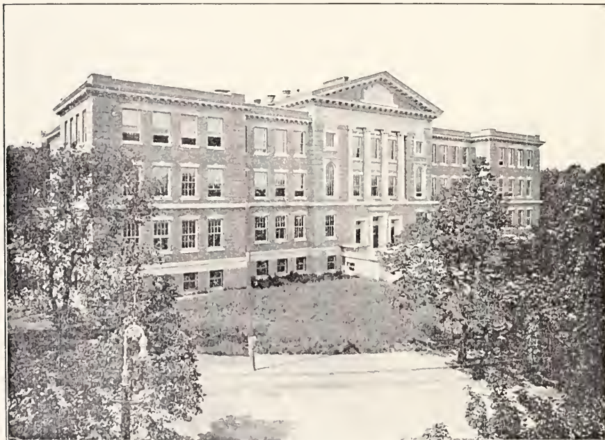
HIGH SCHOOL. Thomas Park, Fronting on G Street.
