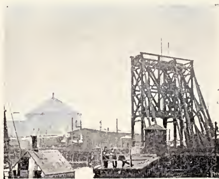
FORMER OLD COLONY RAILROAD BRIDGE.
