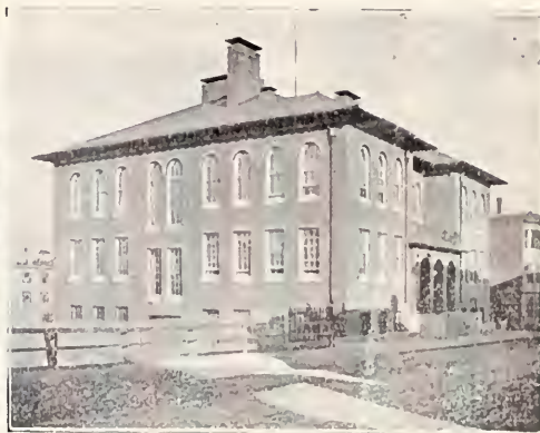
CHOATE BURNHAM PRIMARY SCHOOL East Third Street
