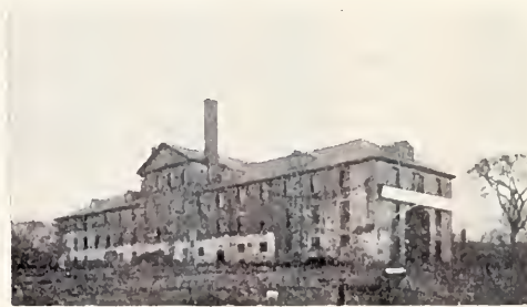
HOUSE OF INDUSTRY. Now used for storage purposes.
