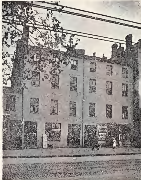
BRINLEY BLOCK. A STREET AND BROADWAY. USED AS A BARRACKS IN 1812.
