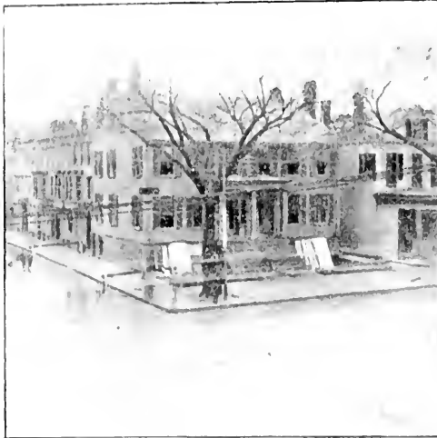
THOMPSON HOUSE, F STREET AND BROADWAY Erected 1840. Demolished 1909.
