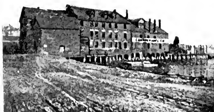
SUFFOLK GLASS WORKS
