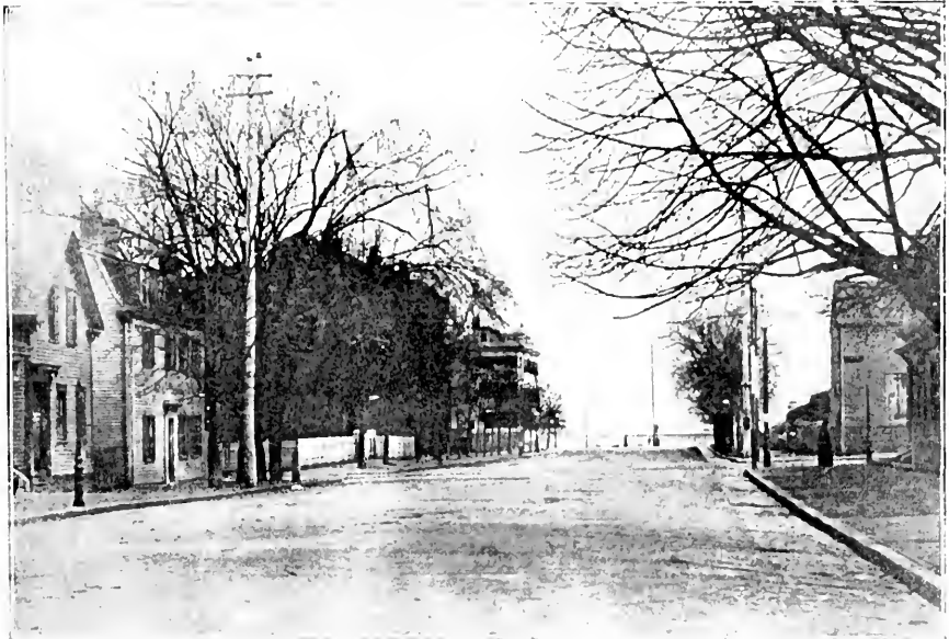
EAST BROADWAY, AT EXTREME POINT (Looking east from O Street)
