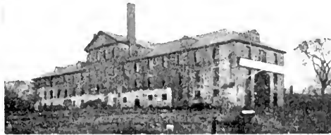
HOUSE OF INDUSTRY. Now used for storage purposes.
