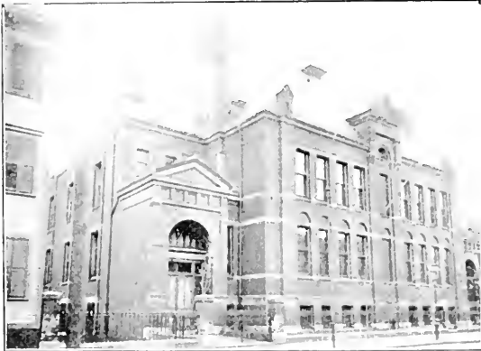
CYRUS ALGER PRIMARY SCHOOL West Seventh Street.
