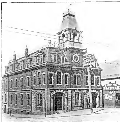
MUNICIPAL COURT Dorchester St Courtroom on corner first floor and Engine Quarters on the right.
