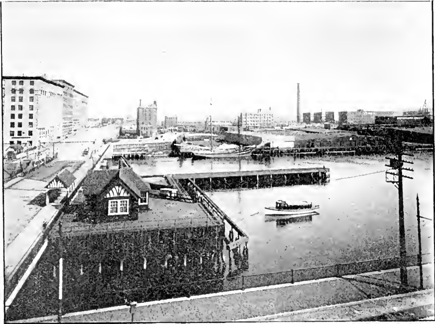
SUMMER STREET EXTENSION BRIDGE. (From roof of South Union Station.)
