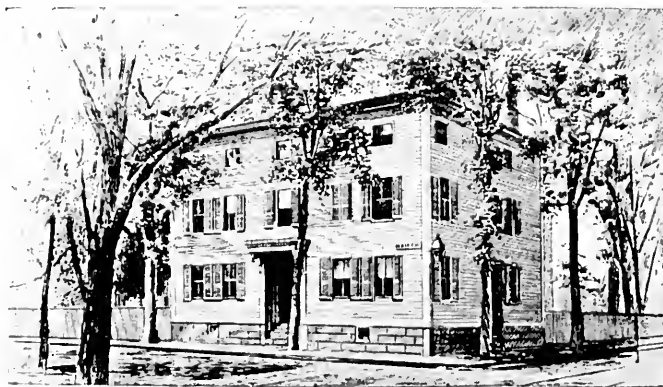
FORMER RESIDENCE OF JOHN HAWES Still standing at corner of Fifth and K Streets.
