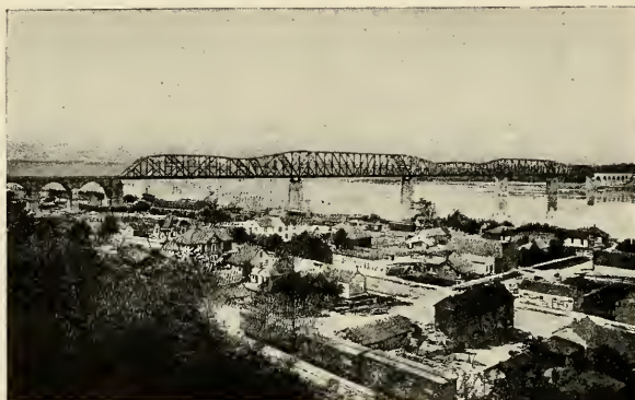
MISSISSIPPI RIVER BRIDGE, THEBES
