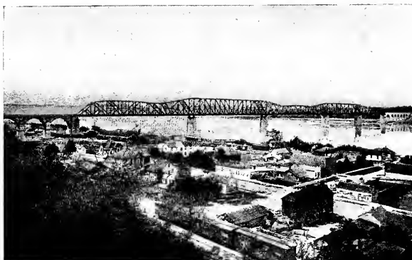
MISSISSIPPI RIVER BRIDGE, THEBES
