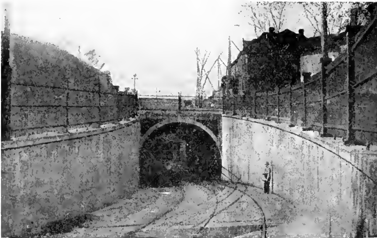
EAST ENTRANCE TO SELBY AVENUE TUNNEL
