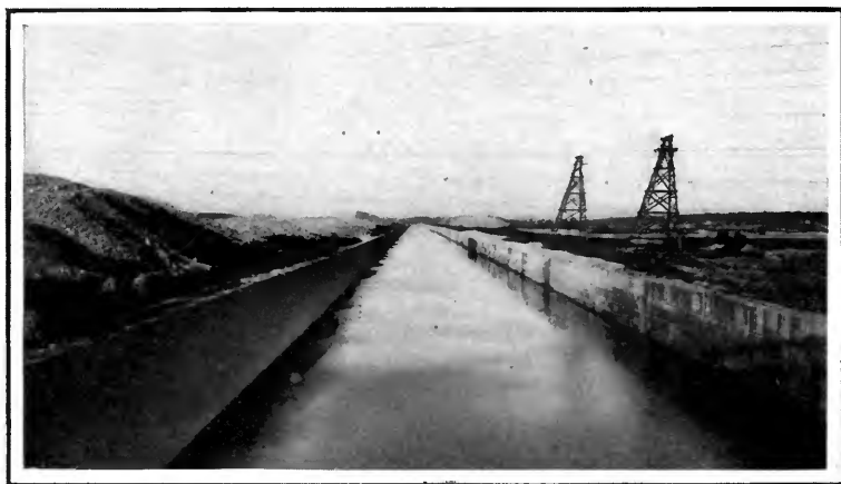
The Drainage Canal—Seventeen Miles of the Canal are Sawed Out of the Solid Rock
