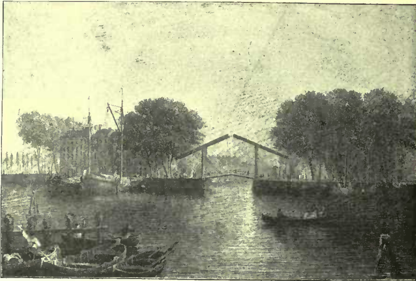
FIG. E. BASCULE BRIDGE ACROSS A DUTCH CANAL.
