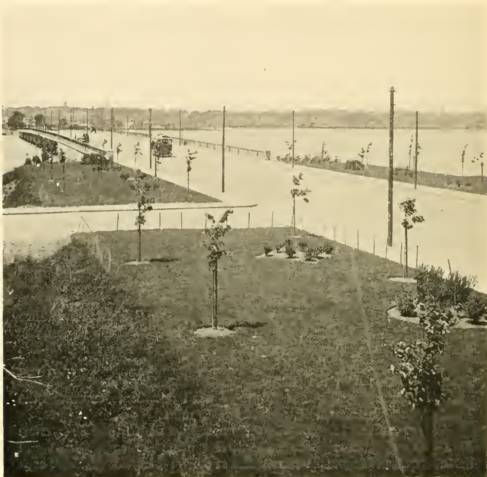
NEW BEDFORD AND FAIRHAVEN BRIDGE
