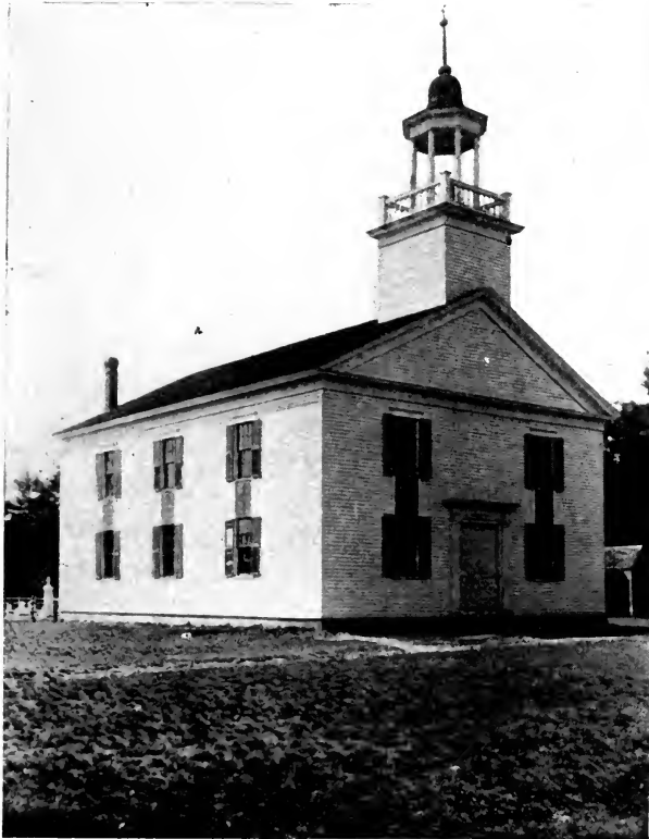
THE BAPTIST CHURCH—BUILT 1824 Centre of Old Home Meetings
