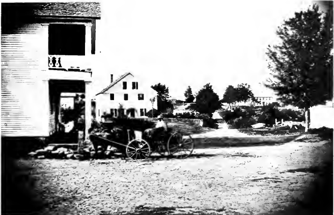
FOUR CORNERS (Looking North).
