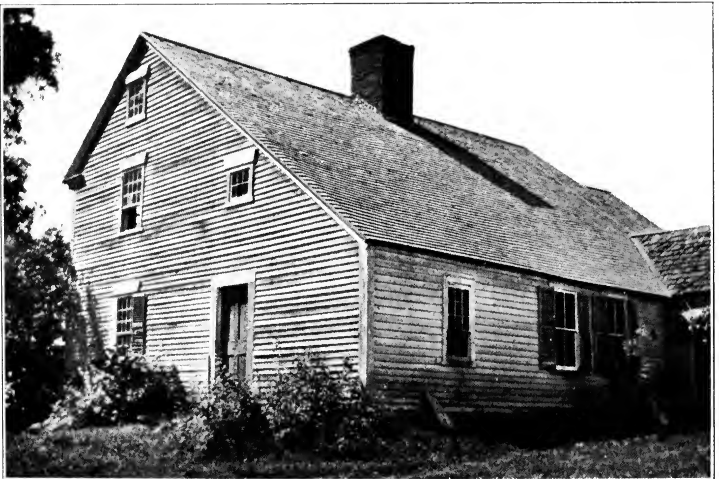
OLD METCALF HOUSE "UNDER THE HILL" Oldest House in Royalston
