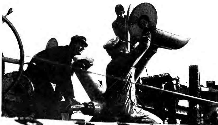
ADJUSTING TIMING MECHANISM ON DEPTH BOMB JUST BEFORE FIRING "Y" GUN
