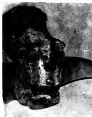
WAR NOSE OF GERMAN TORPEDO FOUND IN FIRE-ROOM OF "MOUNT VERNON"
