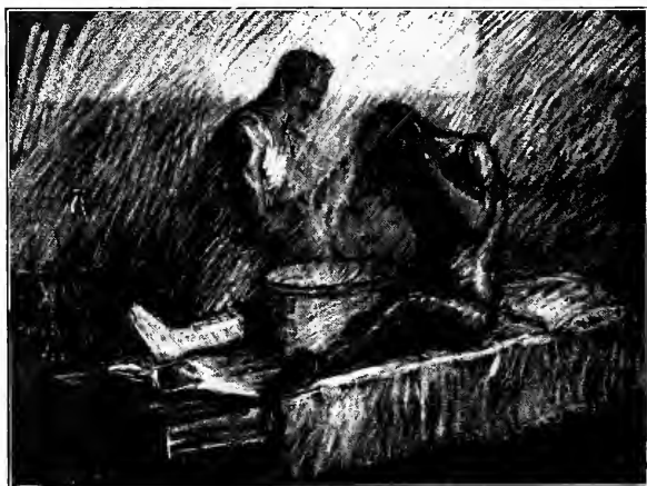
Removing Trench Mud.
