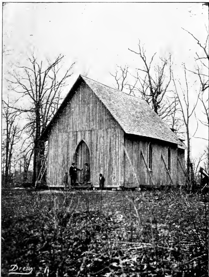
St. Augustines Chapel, erected in 1867, forming part of the enlarged Chapel
