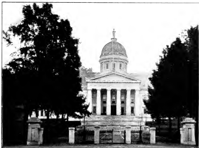
THE PRESENT STATE HOUSE AT MONTPELIER
