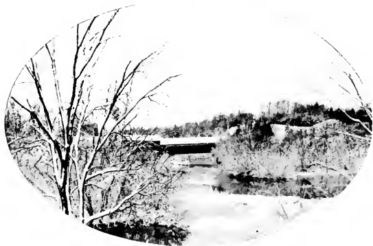
THE BRIDGE TO TINMOUTH IN WINTER.
