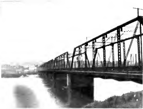
MARKET STREET BRIDGE OVER DES MOINES RIVER, OTTUMWA
