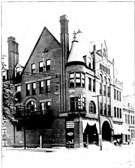
Y. M. C. A. BUILDING, OTTUMWA
