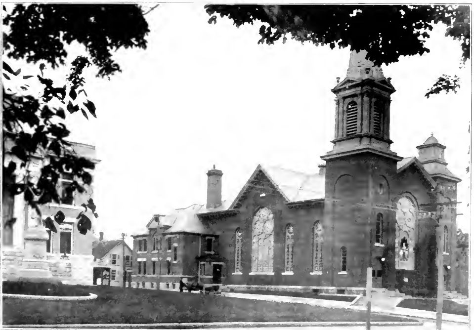
METHODIST EPISCOPAL CHURCH, TORRINGTON
