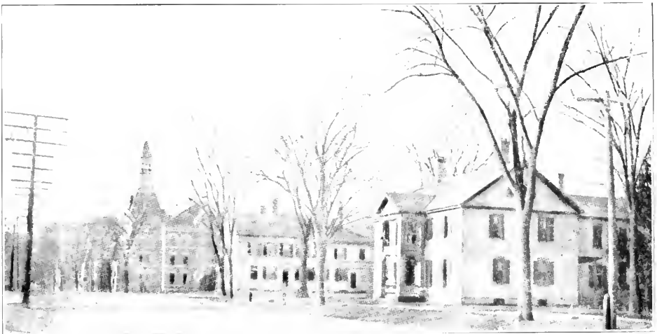
VIEW OF MAIN STREET, THOMASTON
