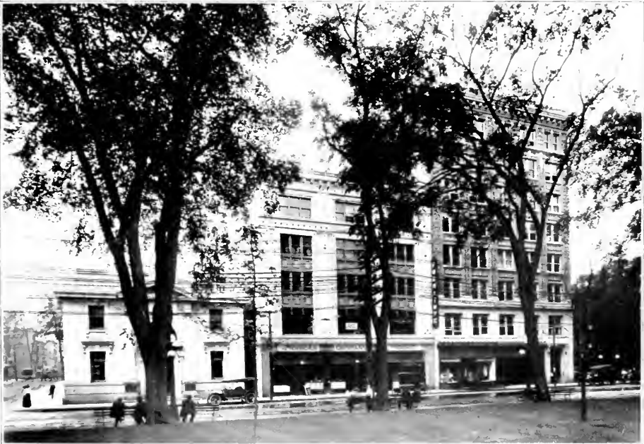
WEST MAIN STREET ARCHITECTURE, WATERBURY From left to right: Colonial Trust Company; Hampson and Lilley Buildings, Viewed from the green.
