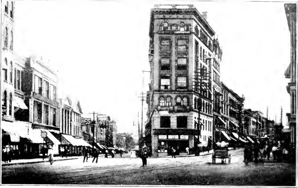
EXCHANGE PLACE, WATERBURY
