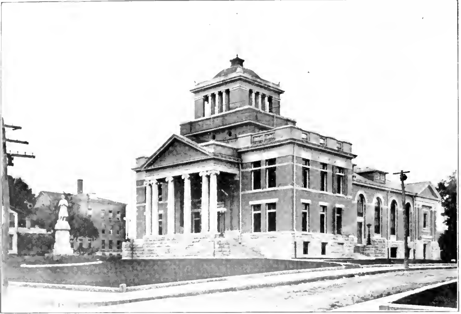
CITY HALL, TORRINGTON
