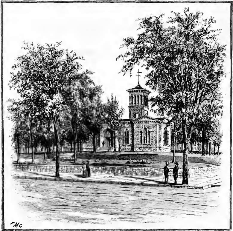
WESTCHESTER COUNTY COURT HOUSE.
