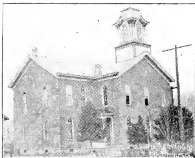
MAGNOLIA HIGH SCHOOL, OLD BUILDING.
