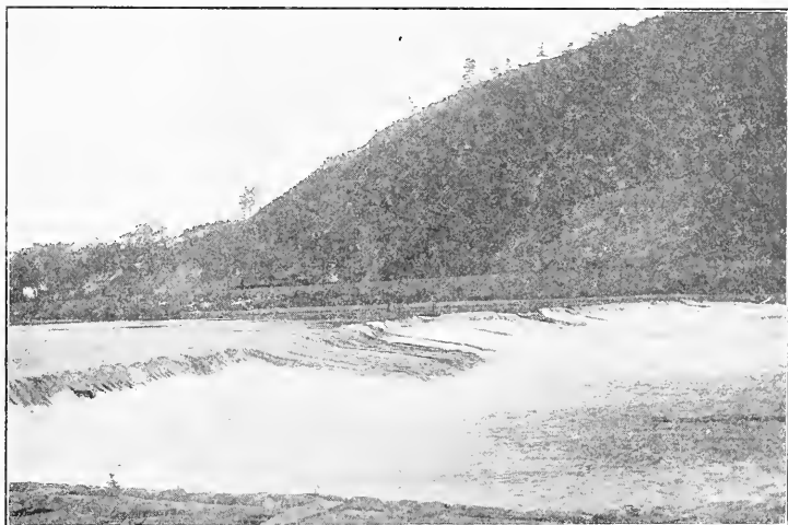
NANTICOKE DAM IN 1899, FROM THE WEST SHORE OF THE RIVER.
