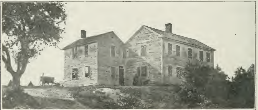
OLD HOUSE ON JOHN HAMMOND PLACE, HIGHLAND STREET. Moved From Site of Present Hammond House When That Was Built.
