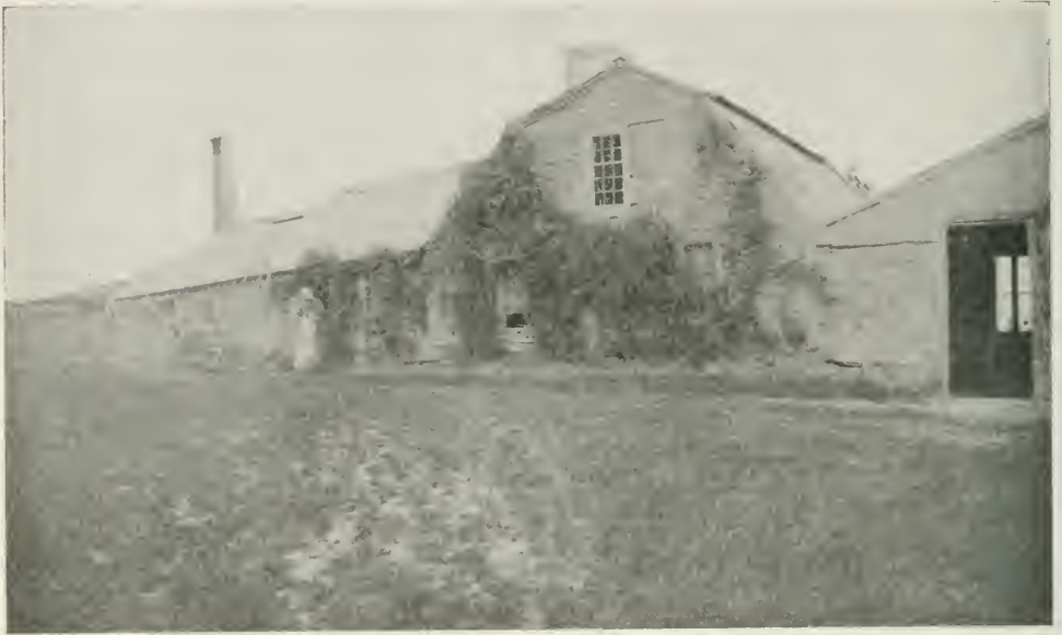
GODDARD HOUSE, HOLDEN ROAD—OLDEST HOUSE IN CITY.
