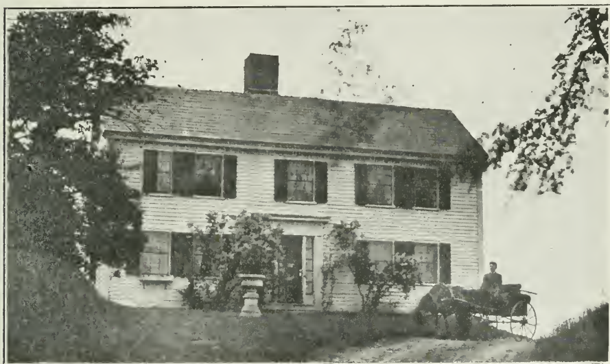
GATES HOUSE, GATES LANE.
