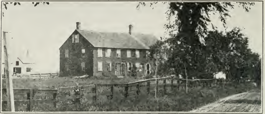
KNIGHT HOUSE, BURNCOAT STREET.
