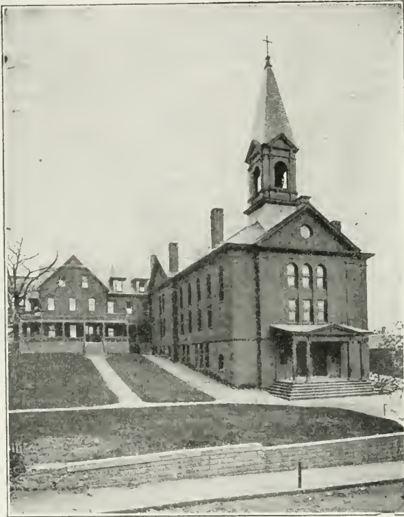
ST. JOSEPH'S CHURCH, WALL STREET.
