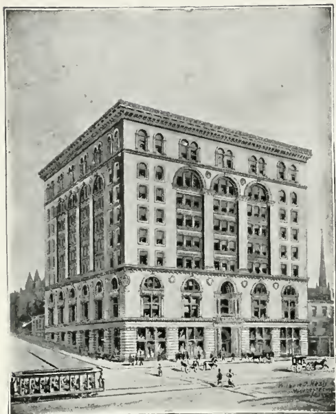
STATE MUTUAL BUILDING.
