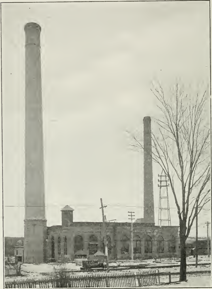
MILLBURY POWER STATION.
