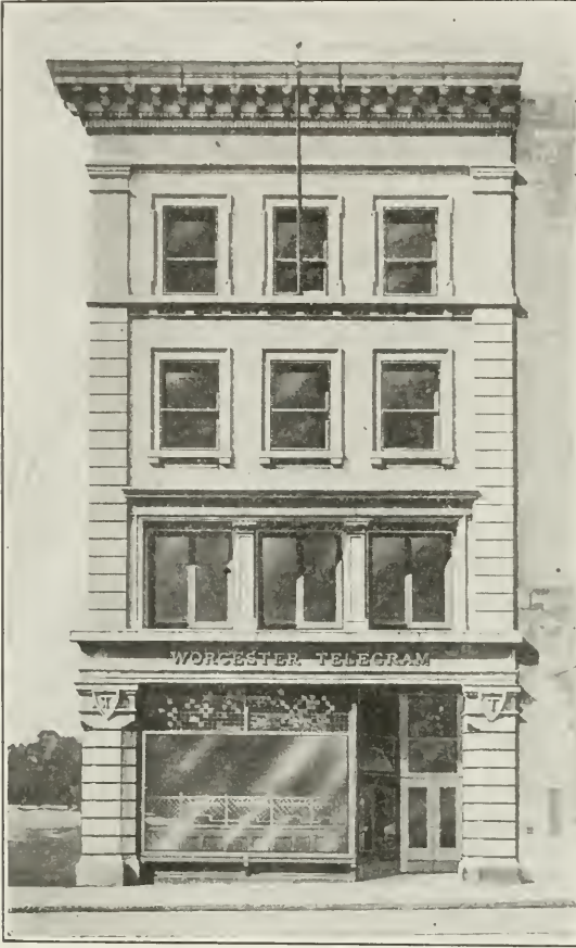
WORCESTER TELEGRAM BUILDING.
