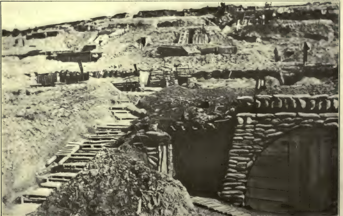
A PANORAMIC VIEW OF THE BURROWS IN WHICH THE DEFENDERS OF VERDUN WERE OBLIGED TO LIVE
