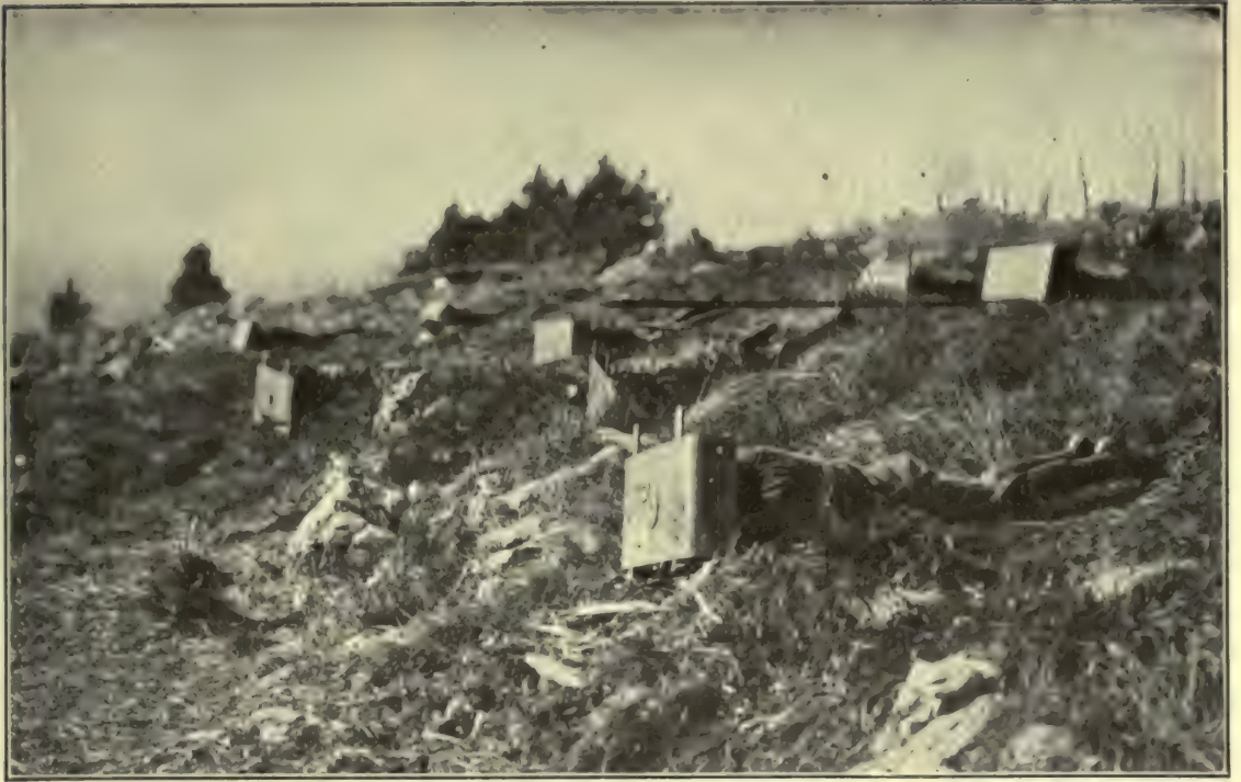
ARMOUR PROTECTION DEVISED FOR THOSE WHO CRAWL FORWARD TO CUT THE ENEMY'S BARBED WIRE
