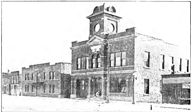
CITY HALL AND ARMORY, EAGLE GROVE.
