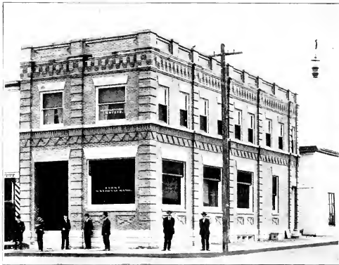
FIRST NATIONAL BANK, KENNEWICK
