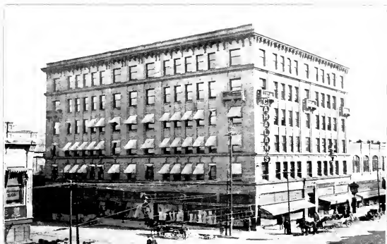
MILLER BUILDING, YAKIMA
