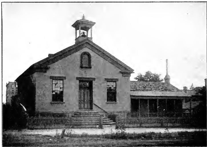
FOURTEENTH WARD ASSEMBLY HALL
