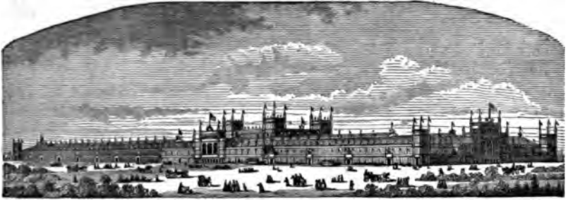
MAIN EXHIBITION BUILDING.
