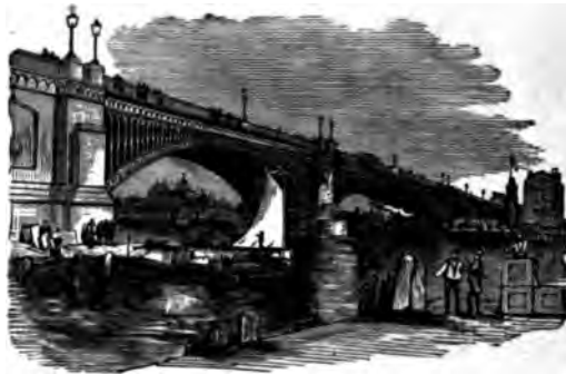
CHESTNUT STREET BRIDGE.
