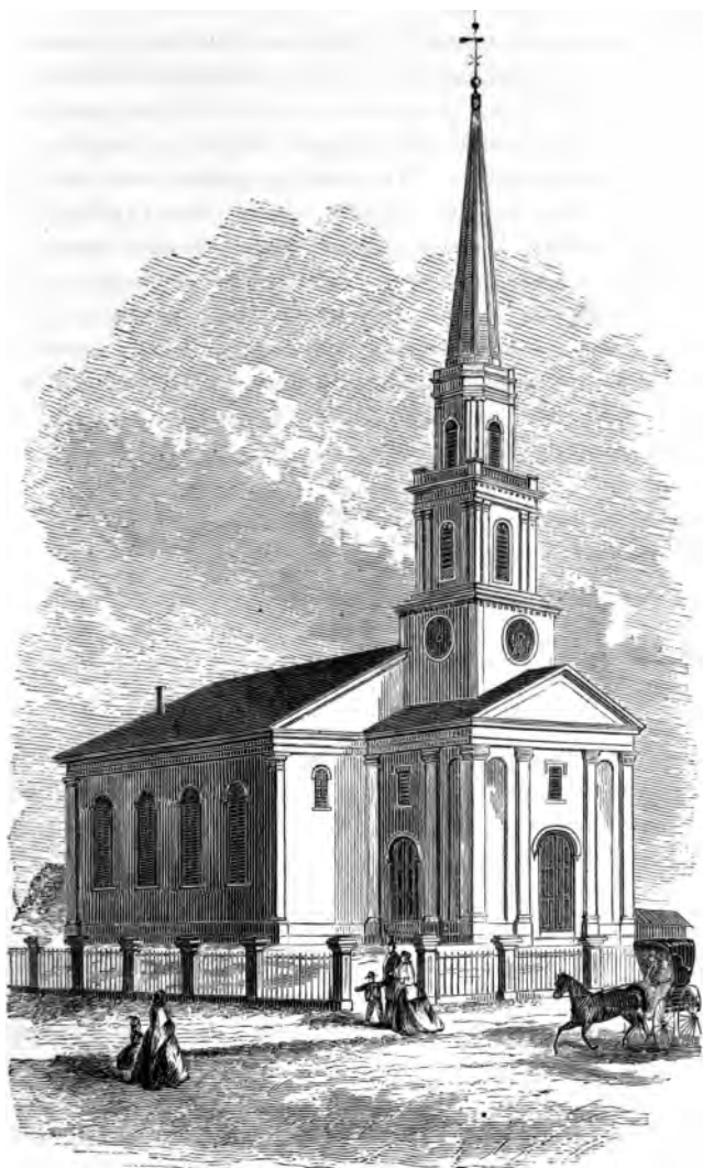
FIRST CONGREGATIONAL CHURCH, CENTRE ABINGTON.
