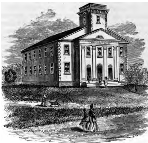
HATHERLY HALL, CENTRE ABINGTON.
