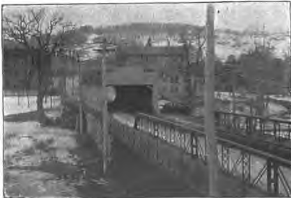
Wooden Bridge at Thomaston, Recently Demolished.
