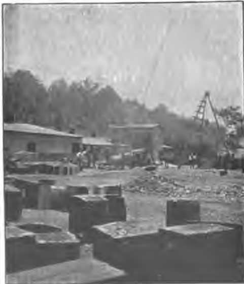
The Old Foundry - Rear View.
