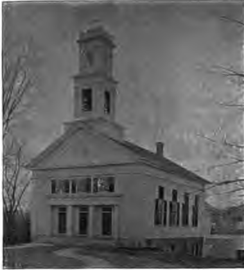
Congregational Church, Terryville.
