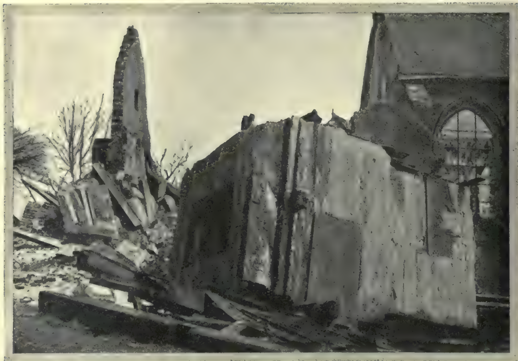
GERMAN OBSERVATION-POST OF CONCRETE, OVERTURNED BY FRENCH ARTILLERY.
