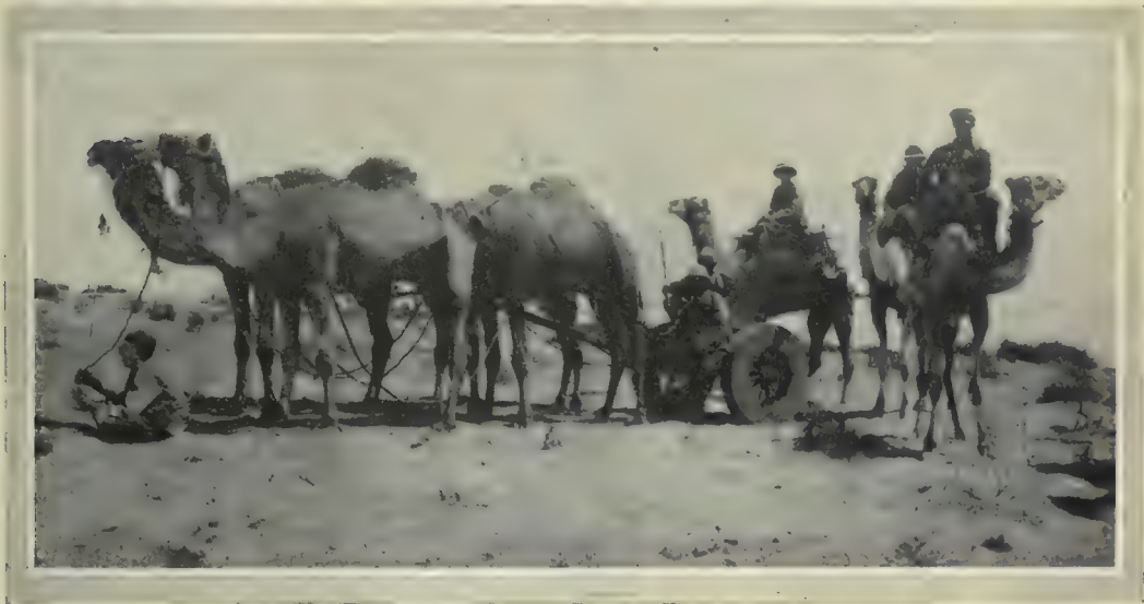
CAMEL TEAM DRAWING A CABLE-LAYING CHARIOT.
