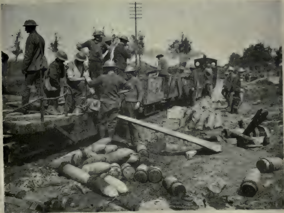
LOADING SHELLS ON A LIGHT RAILWAY.
