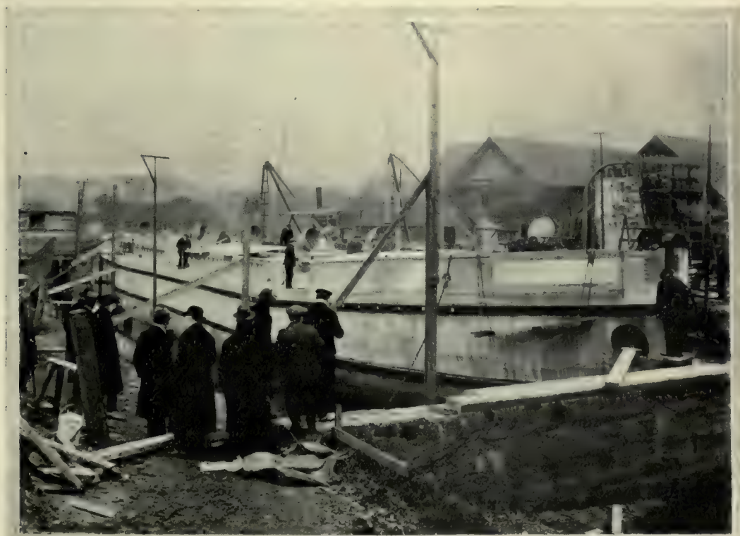
A CONCRETE SHIP NEARING COMPLETION.
