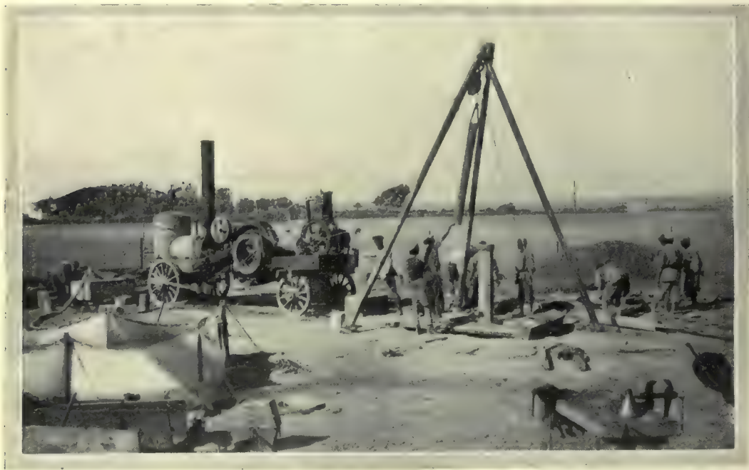
ENGINEERS BORING FOR WATER.
