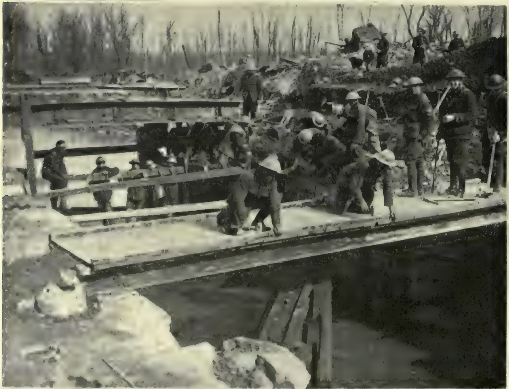
REPAIRING A LOCK.
