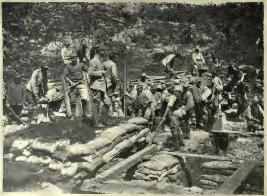
ITALIAN SOLDIERS REPAIRING A BOMB-PROOF SHELTER AFTER BOMBARDMENT.
