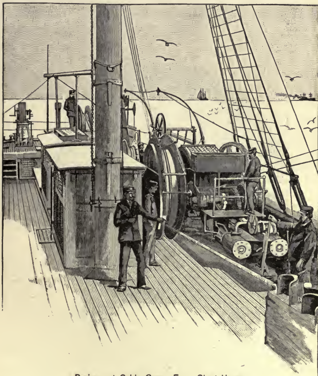
Paying out Cable Gear. From Chart House.
