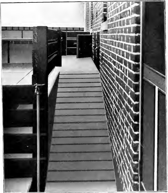
Fig. 13—Hog Entrance to Operating Rooms.
