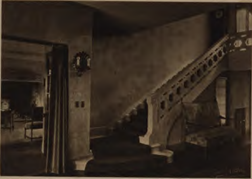
A Main Hall Staircase in Concrete
