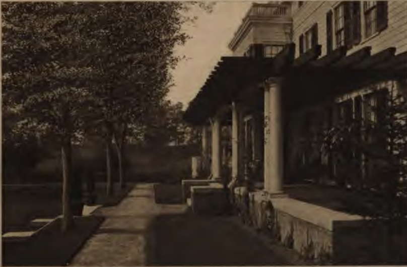
A Delightful Porch on Residence in Greenwich, Conn.
