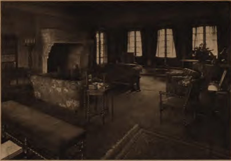
Another View of the Fireproof Interior Shown on Opposite Page
