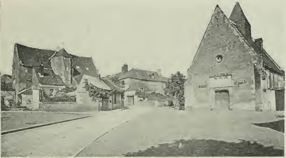
THE CHURCH AND THE HOUSE OF THE PAGES OF FRANCIS I. AT CHENONCEAU. NO RULE COULD BETTER ITS ACCIDENTAL COMPOSITION
