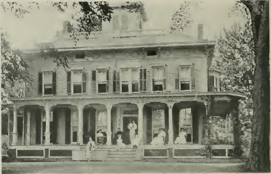
THE OLD BOWNE HOUSE AT TENAFLY BEFORE IT WAS REDESIGNED.
