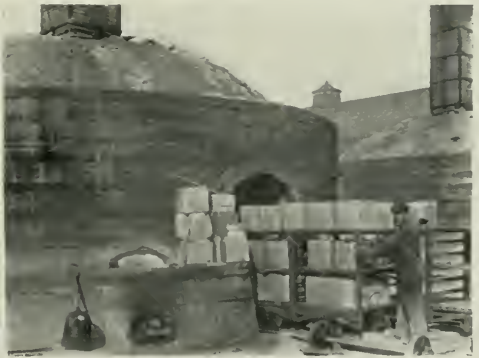
FIGS. 3 and 4. WHERE THE CLAY BLOCK IS DRIED AND BURNED.
