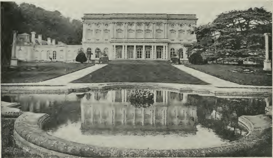
THE EAST FACADE.
