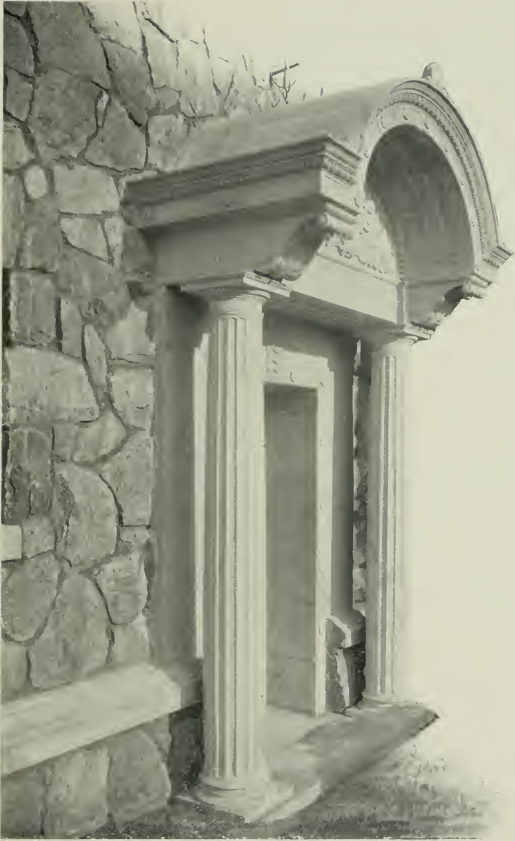
THE ENTRANCE TO THE LIBRARY AT VYGERBERG FARM IS AN EXAMPLE OF ADVANCED CONCRETE CONSTRUCTION.
