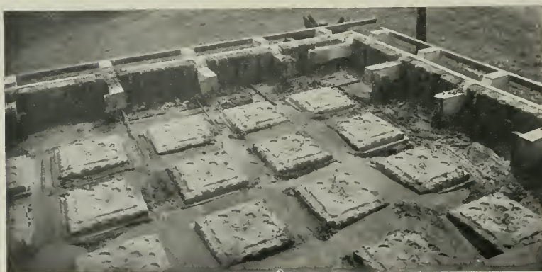
FIG. 15. THE CONCRETE PARTLY POURED.
