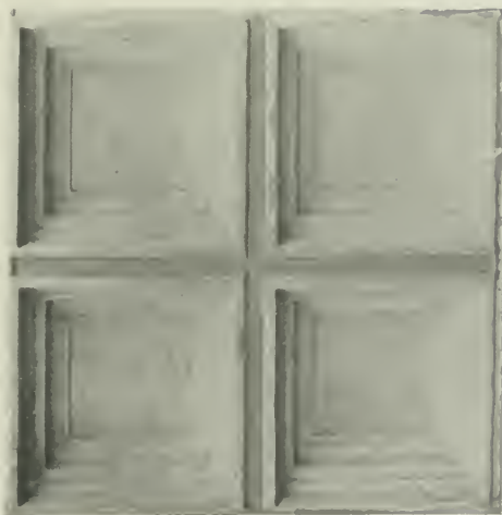
FIGS. 17 AND 18. CONCRETE CEILINGS CAST OVER SAND MOULDS.
