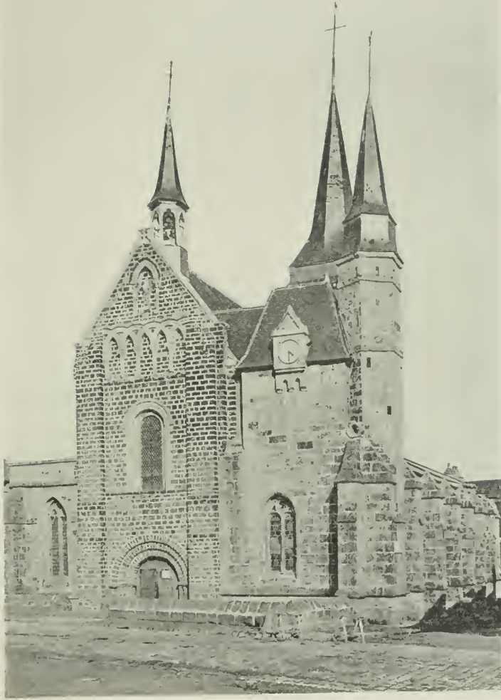
THE NAVE OF THIS OLD CHURCH AT BROGLIE IS BUILT OF STONE NOW USED FOR THE THIRD OR FOURTH TIME AND CUT DOWN IN SIZE BY EACH REFITTING. IT IS NOW HALF WAY BETWEEN BRICK AND STONE AND HAS JUST THE SCALE OF TEXTURE TILE.
