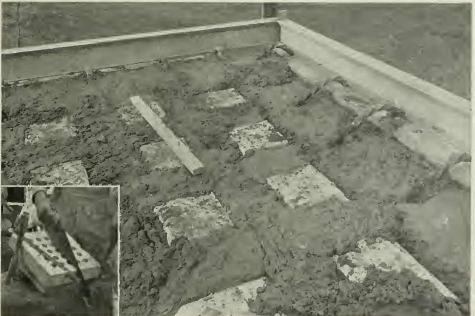
FIG. 33. THE NEARLY COMPLETED SLAB.
