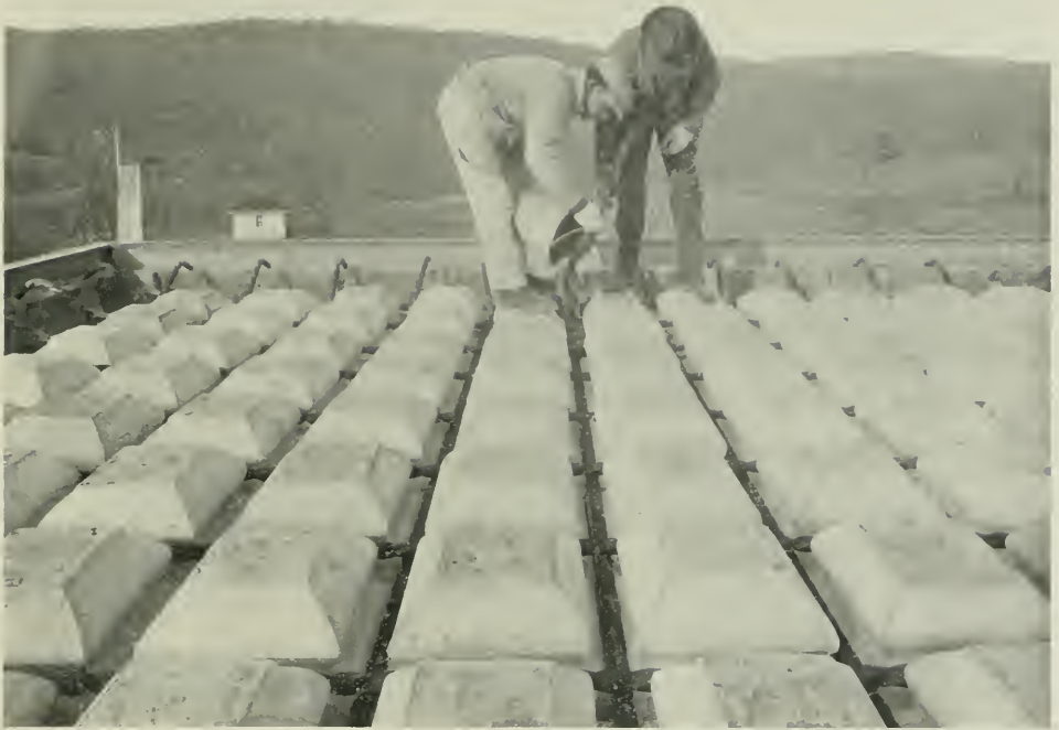
FIG. 32. THE REINFORCEMENT IN PLACE.
