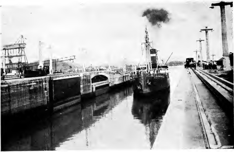
The first steamer to enter the Panama Canal.
