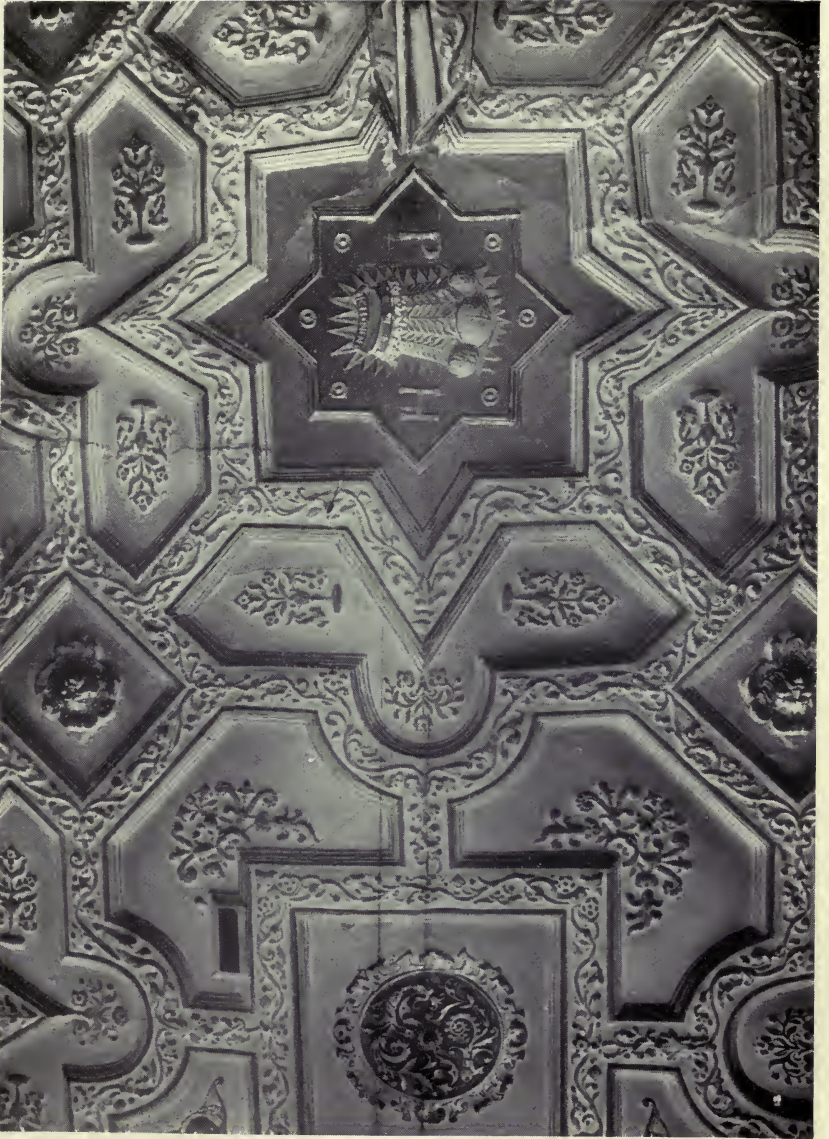
No. 17, Fleet Street; ceiling of room on first floor.
