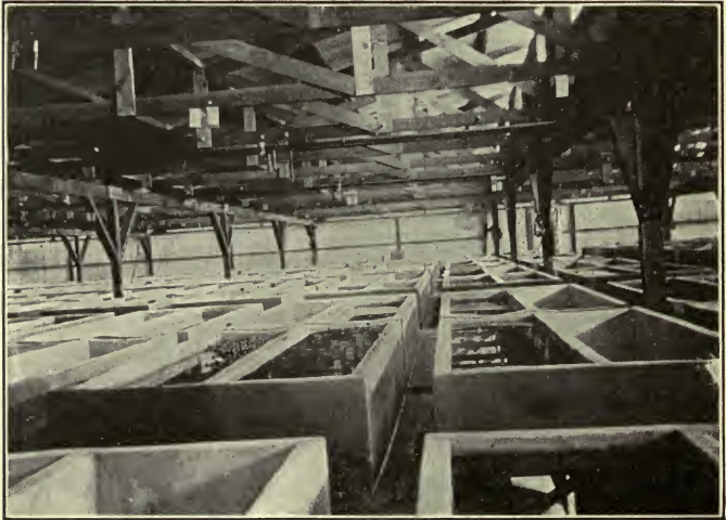
FIG. 55. Interior of Large Olive Pickling Plant.
