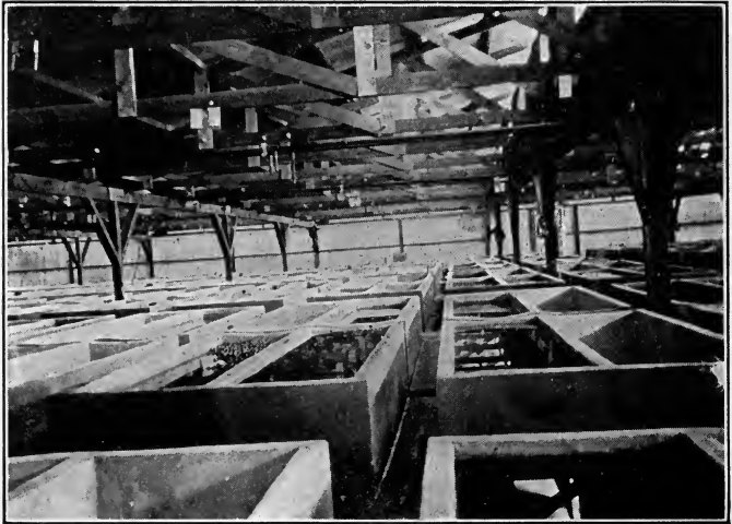
FIG. 55. Interior of Large Olive Pickling Plant.
